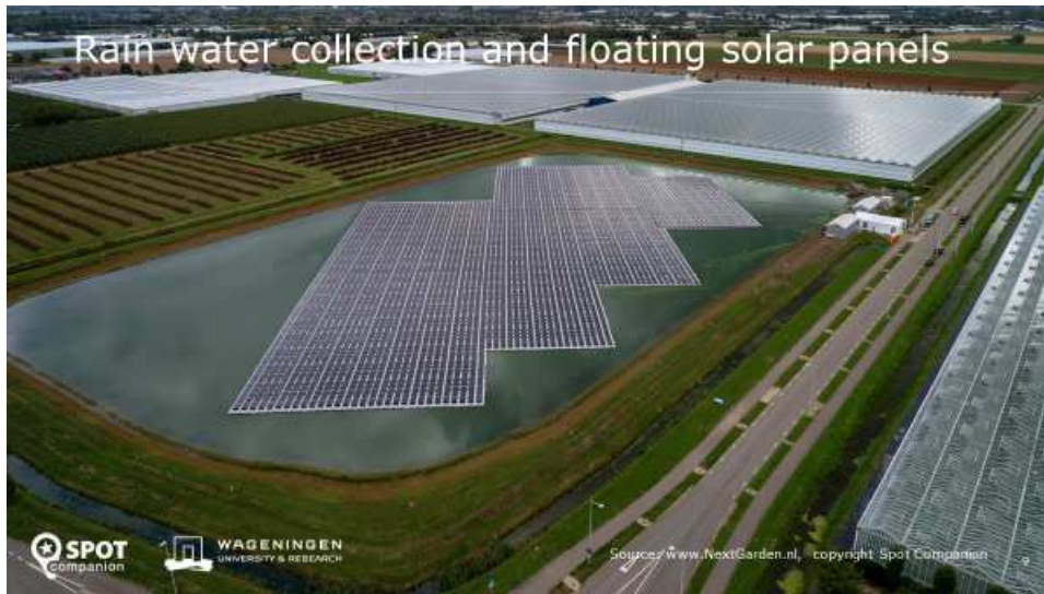
Figure 4.7 Rainwater collection and floating solar panels in NEXTgarden (NL). Photo © SPOTCompanion.
